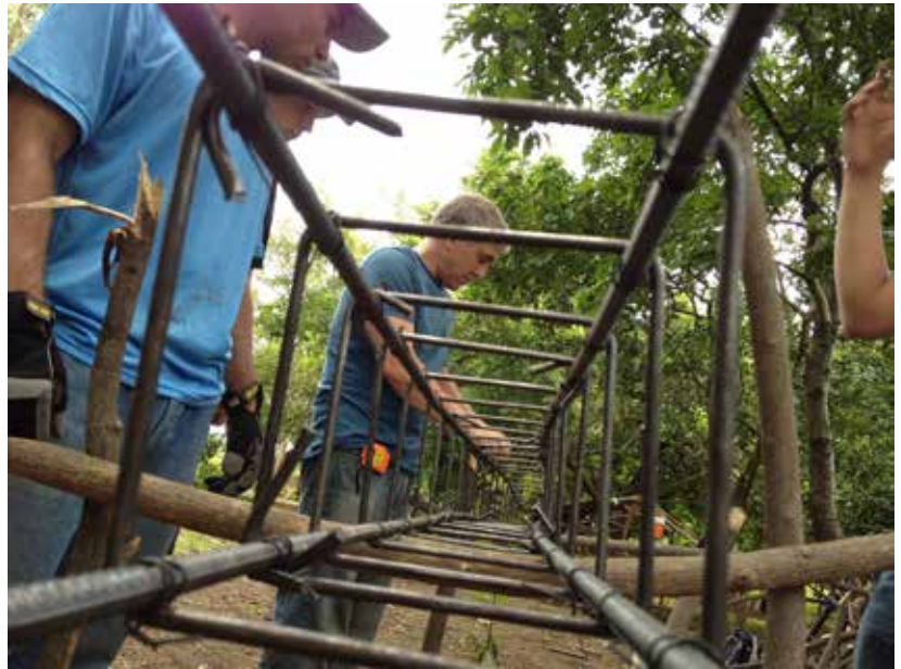
Seth Wachtel (center) tying steel in Nicaragua.
